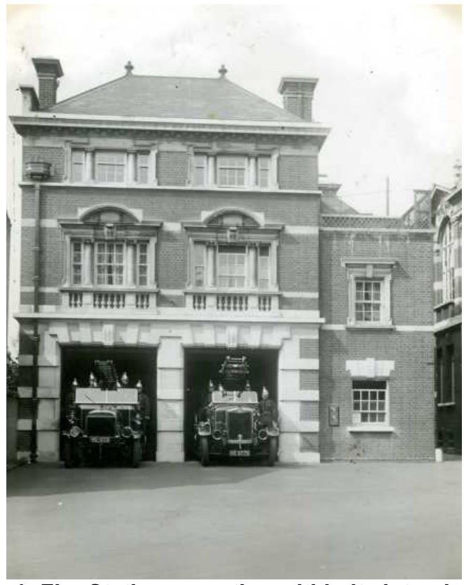
Photo 1: Fire Station operating within its intended use
